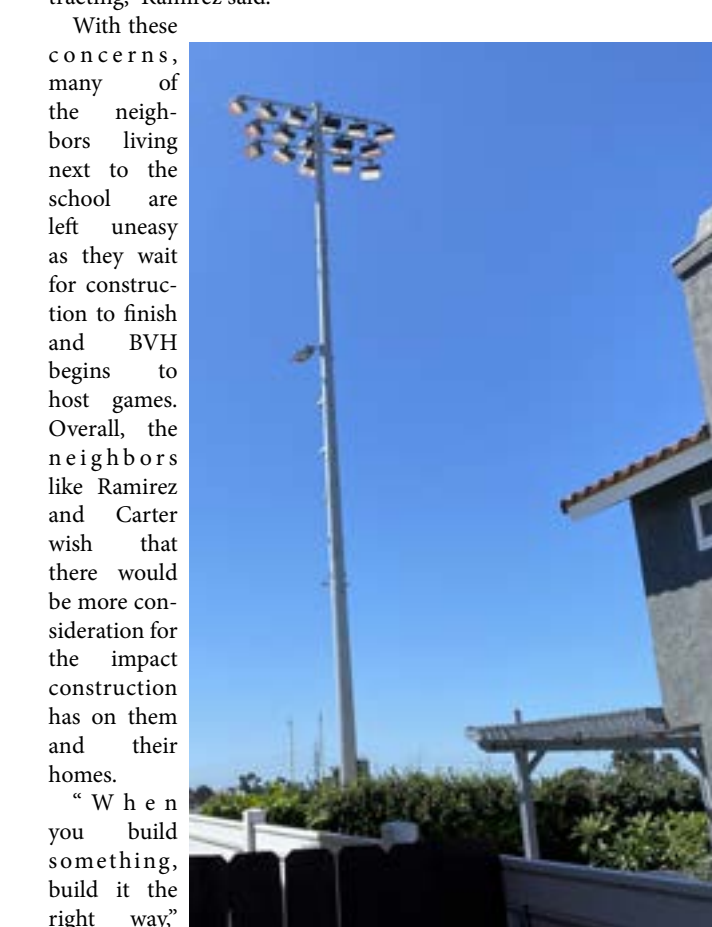
View of one of the floodlights that is directly behind the neighbors backyard that live next to the field. Some neighbors have complained that it shines on their property and is very bright. PHOTO TAKEN BY ANGELINA RUCKMAN
